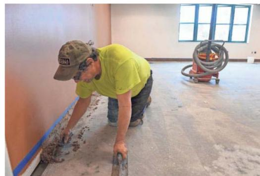
**Robert Hensel, of Plexi-Chemie Inc., starts work on a high performance seamless epoxy flooring being installed in one of eight new classrooms on April 17 in the new 14,000-square-foot addition being built.**
